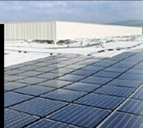
Rooftop Solar Array
